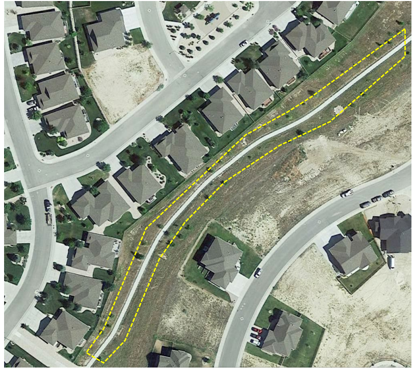
Figure 13. New housing construction that required the installation of a separate multiuse pathway throughout the neighborhood. This particular path opened onto the backyards of homes into a natural ravine, giving residents quick and safe access to the trail. See PI-2.
